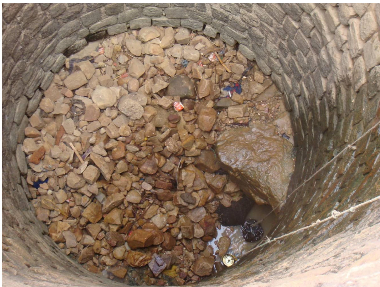
Well in Koyra, February
