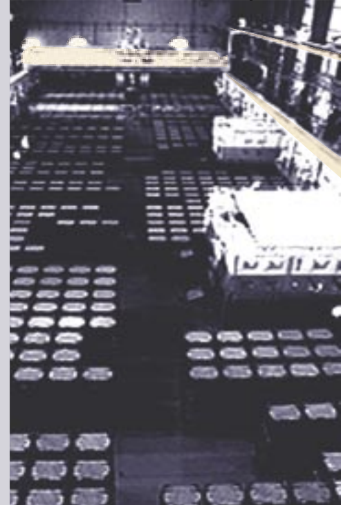
Storage pond in thermal oxide reprocessing plant, Sellafield, United Kingdom
